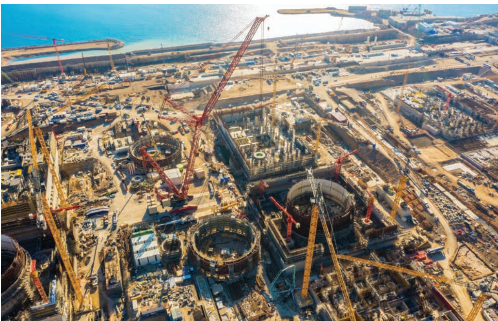
Unit 3 under construction (Image: Akkuyu NPP)
