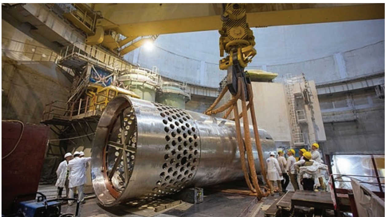
Work to install Rooppur 1's core barrel was completed in May 2023 (Image: Rosatom)
