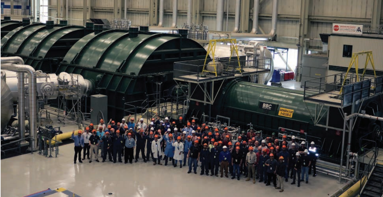
U3 Returned to Service – staff on the Turbine floor photo (Image: OPG)
